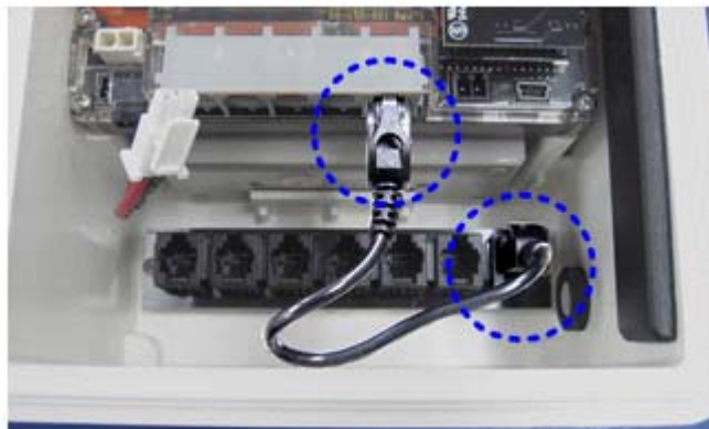
Figure 32: Figure 30: Installing Connector Cable
