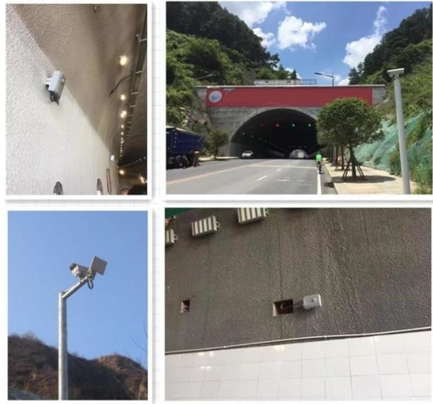
and flame retardant polycarbonate to achieve an IP67 / NEMA 4X protection rating. The AO- LXP21E is able it to withstand the corrosive atmosphere and regular tunnel washing that the tunnel environment endures. The AO-LXP21E has an operating temperature range from -30°C - +70°C which ensures stable readings across all prevailing ambient temperature conditions.
